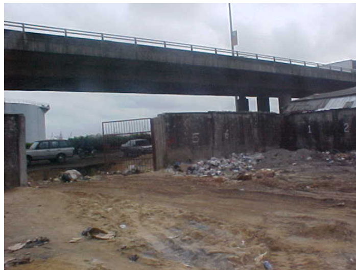
Plate 1. Temporary car park access.
