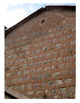
**Figure 22.** Combination of brick and stone (alternative wall) in a dwelling wall in Bergama (Ancient Pergamon), western Turkey, (Construction date: early 20<sup>th</sup> century, photograph by Kavas (2012).
