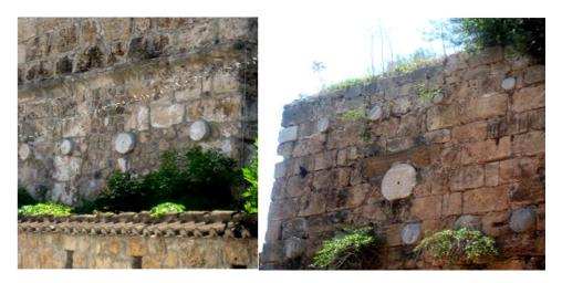
**Figure 16.** (Left) a general view of the spolia columns vertically integrated to masonry. (Right) spolia columns with changing diameters integrated to the fortifications of the citadel of Antalya (Attaleia), southwestern Turkey (Construction date: Anatolian-Seljuk period, early 13<sup>th</sup> century / photograph by Kavas (2012).
