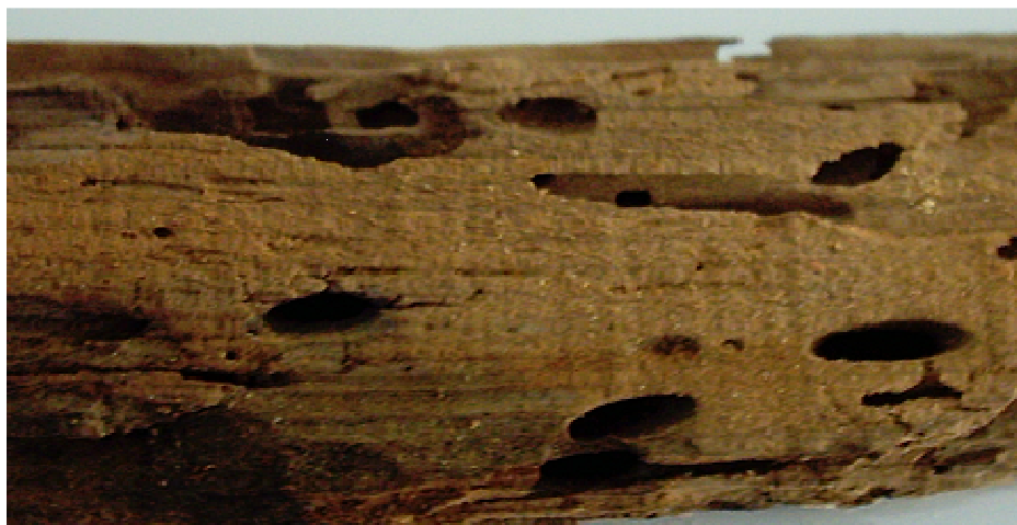
Figure 2. Damage of L. brunneus (Steph.).
